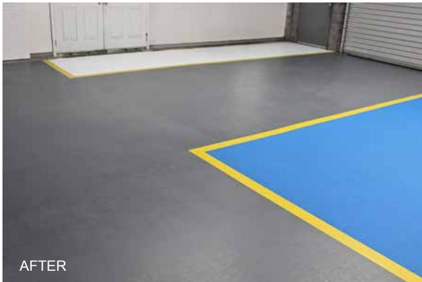
After repairing and grinding the floor, DiamoPro Diama-TLC was applied to demarcate traffic (gray), work (blue) and equipment (white) areas. The lithium colorant hides repairs and restores a uniform tone to the floor. DiamoPro UV HS was used as a topcoat to ensure years of abrasion and stain resistance.
