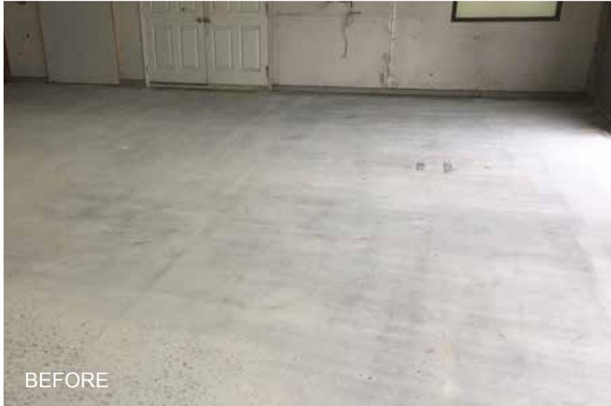
This concrete floor in a warehousing and service facility exhibits typical symptoms of years of wear. Cracks, spalls and pitting appear over much of the surface area, along with oil, grease and solvent stains. The floor has been marred with skid marks, ground-in abrasion, and discoloration from heavy equipment traffic.
