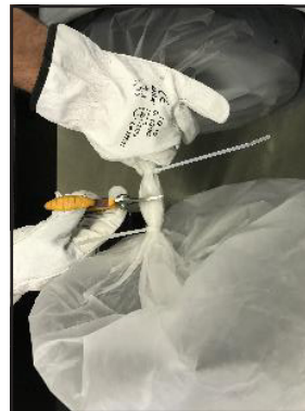
2 - Cut the strip between the two bands.
