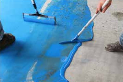
Roll TLC in a thin coat. Let coat dry for one hour. Reapply coats depending on the color intensity desired.
