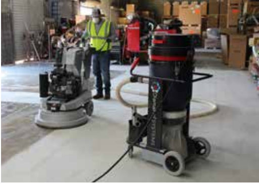
Grind floor to a 120 grit finish.
